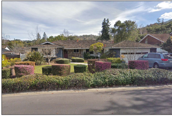
The Site and existing house
